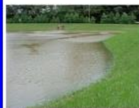
Extended Detention Basin - full.
